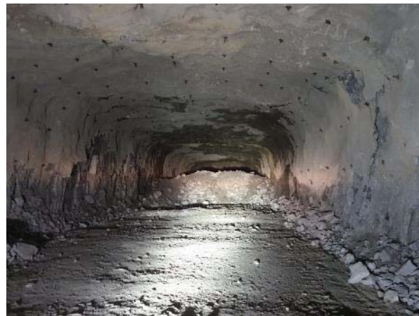
Figure 4: Rock bolts installed in Grapenberg mine and view of a drift.
