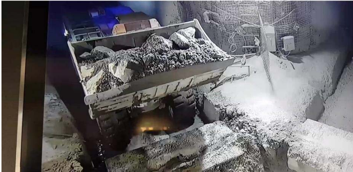
Figure 24: Loader at a dumping shaft.
