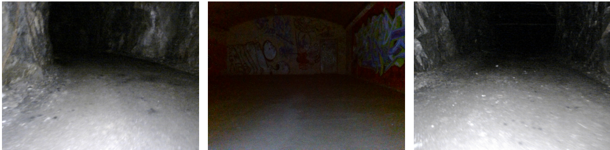
Fig. 7: The images from the looking forward camera of the MAV navigation in three different environments of an underground tunnels in Sweden.
